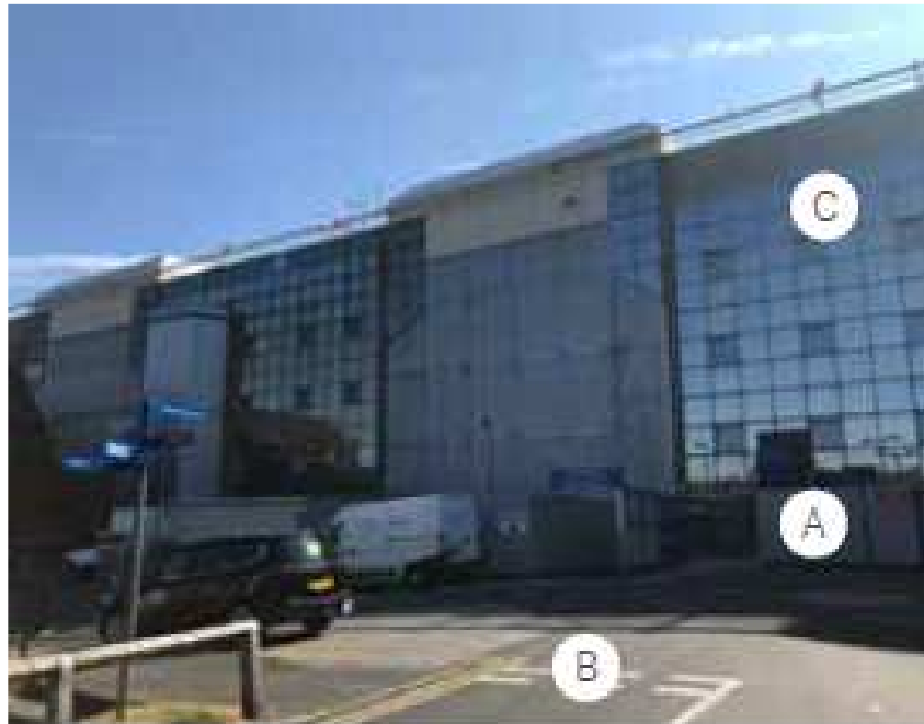
05. VIEW OF EXISTING HOSPITAL FACADE
